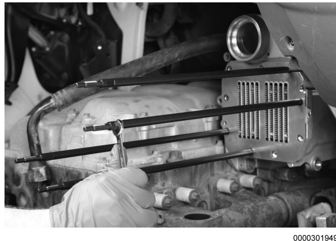
Figure 3. Threaded Rod Tightening.
